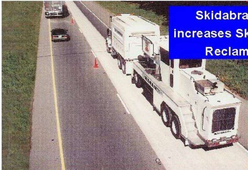
Skidabrading the surface increases Skid Numbers Prior to Reclamite Application
