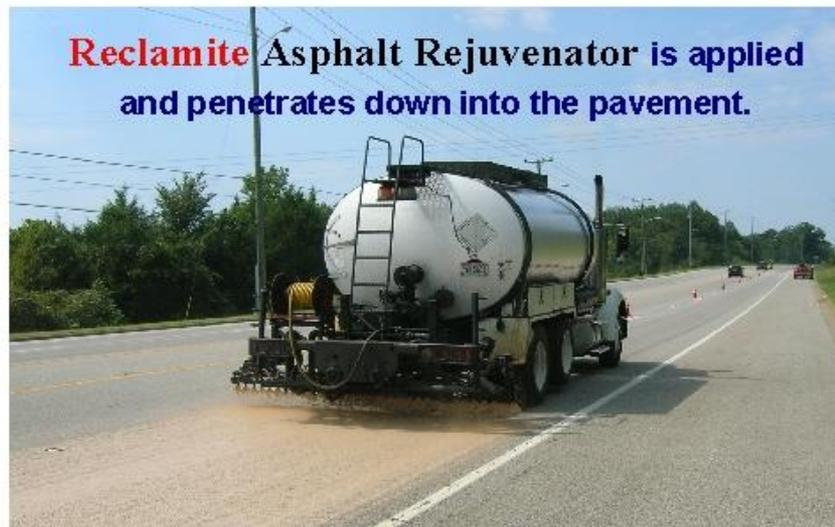
Reclamite Asphalt Rejuvenator is applied and penetrates down into the pavement.
